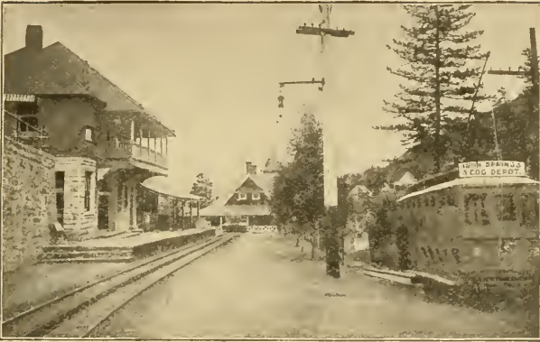
COG ROAD STATION, MANITOU
